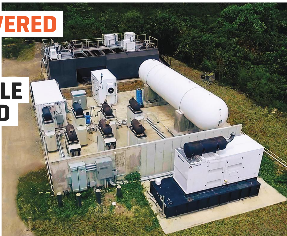
The Magens Junction microgrid is powered by seven propane-fueled microturbines. The 18,000-gallon on-site propane storage tank provides eight to 10 weeks of fuel autonomy before a refill becomes necessary. [Images courtesy of Capstone Green Energy.]
