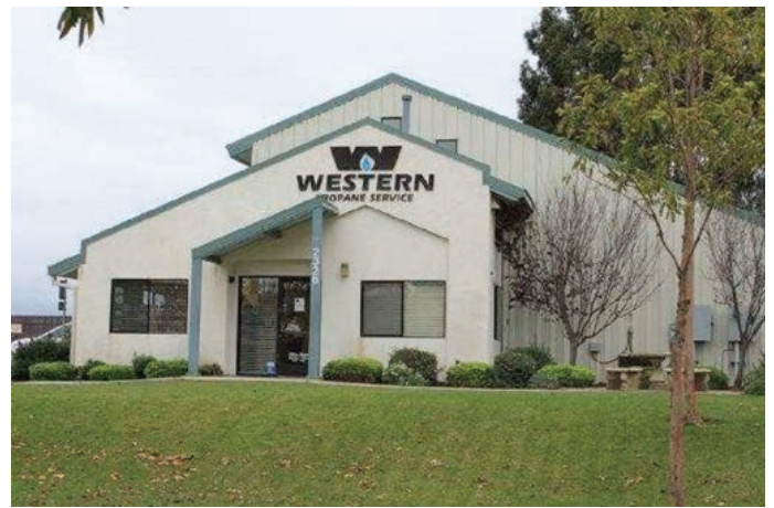
The Western Propane headquarters in Santa Maria, Calif., was built in 2000.
